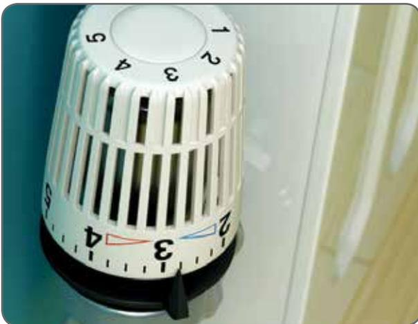
**Never turn the radiator valves tightly off,** as this can cause them to jam. As a general rule, setting the radiator valve to the middle setting will produce a comfortable temperature. Turning the radiator valve higher will not make the room heat up more quickly; it will lead to the radiator continuing to heat the room beyond the temperature you need, making it uncomfortably hot and wasting energy.
